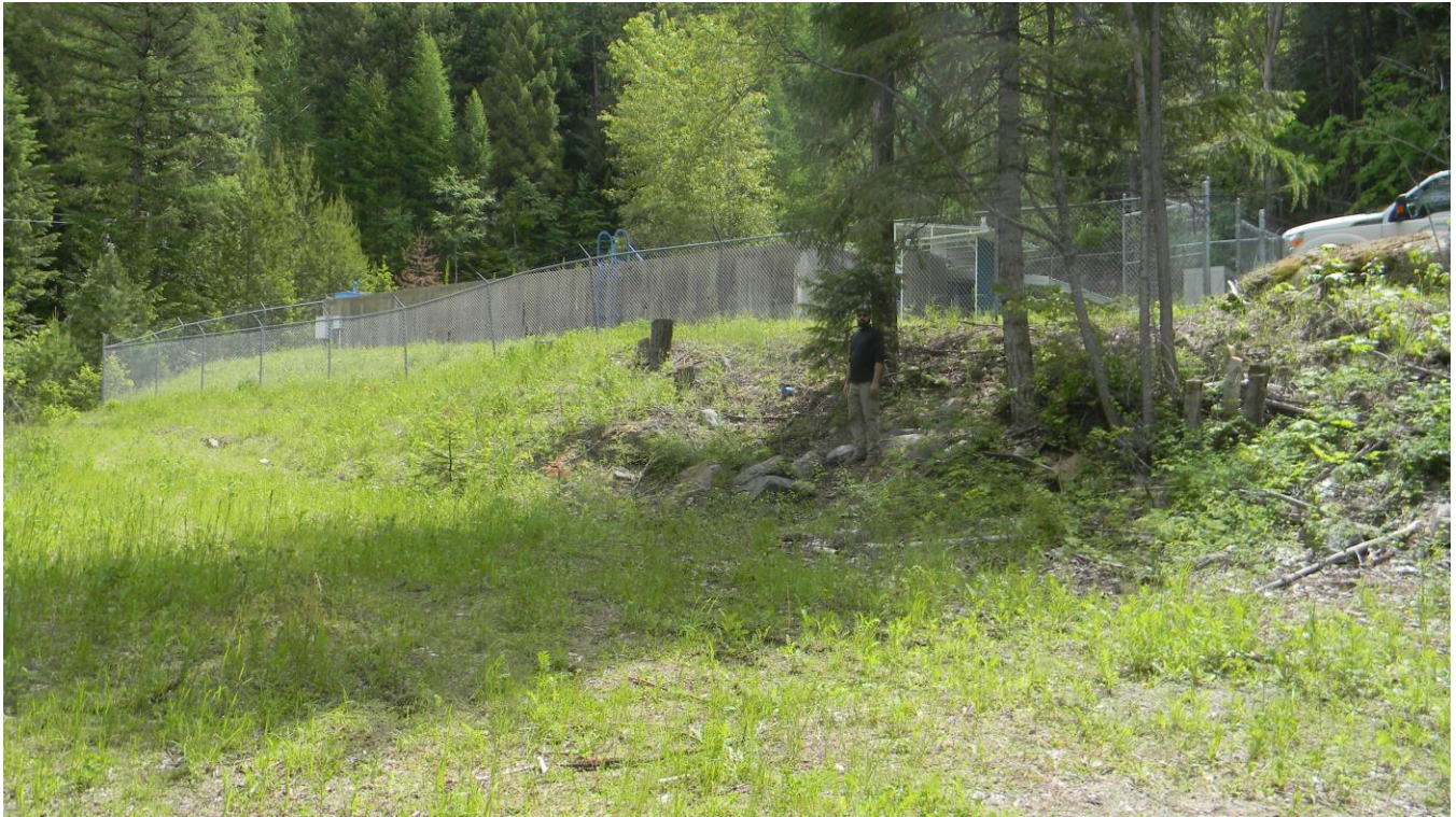
Figure 18. Photograph of the Cabinet Mountain Water District Project area taken at the existing Black Mountain Tank and Booster Station. Jeremy Davy is standing at the drainage outlet that may be improved in the future. The view is to the southeast.
