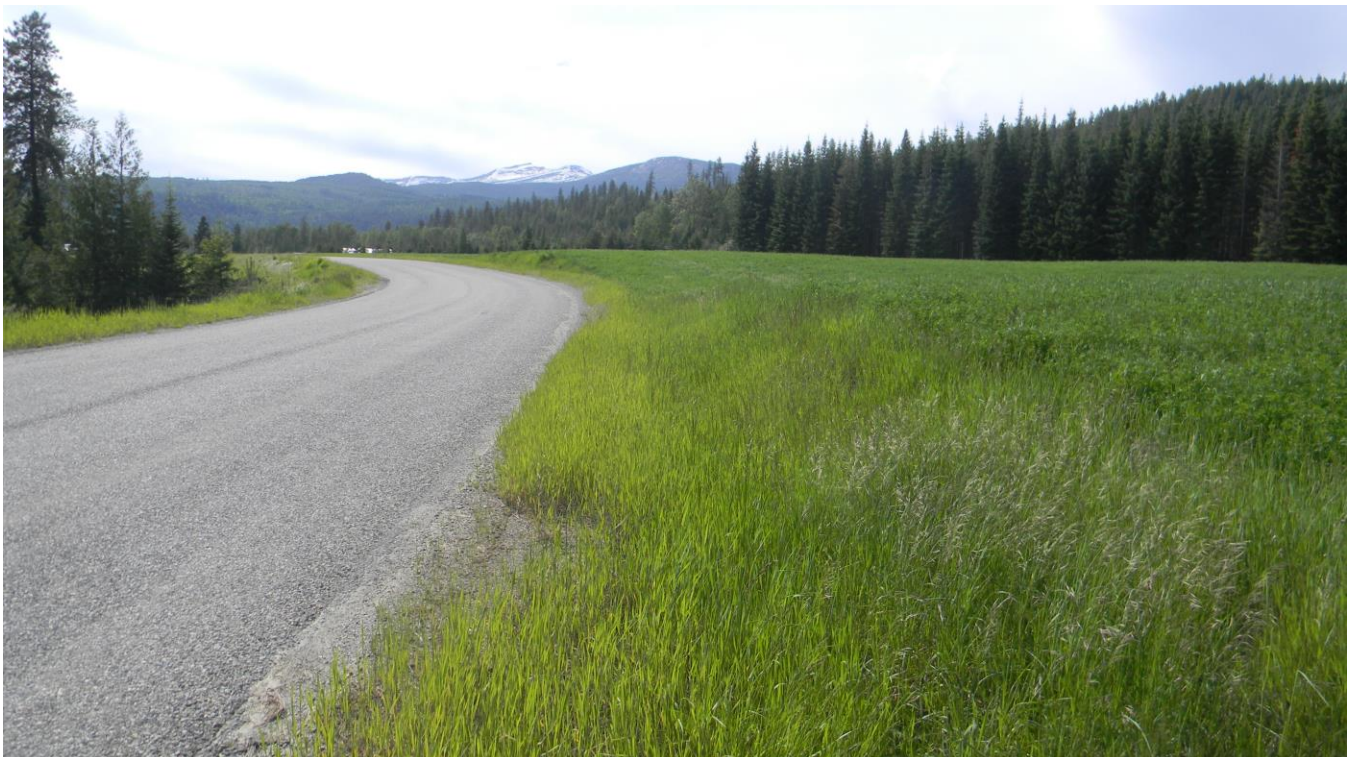
Figure 37. Photograph of the Cabinet Mountain Water District Project taken along the waterline route between the Highland Booster Station and access road to the new Highland Tank. Highland Flats Road is at the left. The view is to the west.
