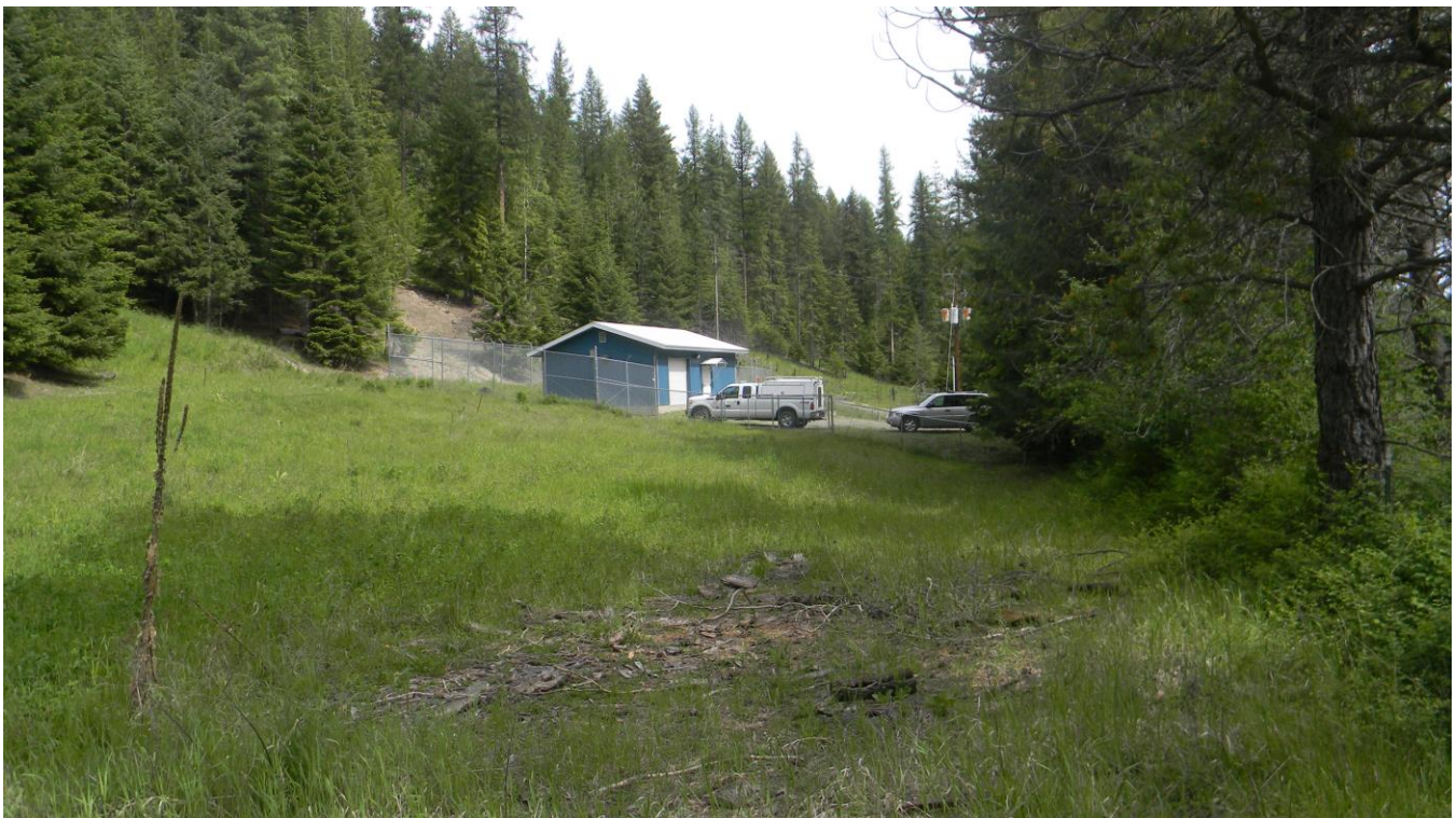
Figure 11. Photograph of the Cabinet Mountain Water District Project area taken south of the Parker Canyon booster station. Most of the new property is visible in the foreground and center of the photograph; the new tank will be constructed at the base of the hillside to the left of building. The view is to the northwest.
