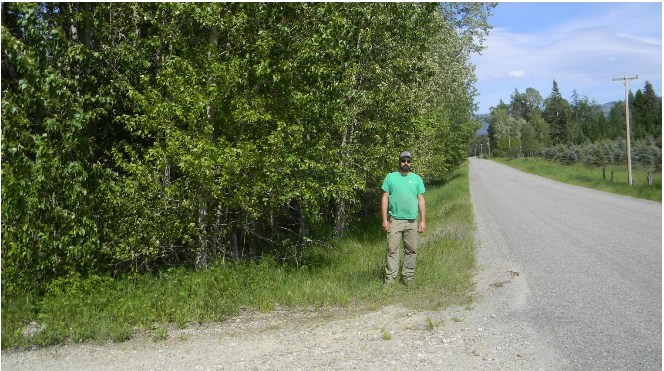
Figure 41. Photograph of the Cabinet Mountain Water District Project taken along the waterline route between the Highland Booster Station and the access road to the new Highland Tank (in the foreground). Highland Flats Road is at the right. The view is to the east.
