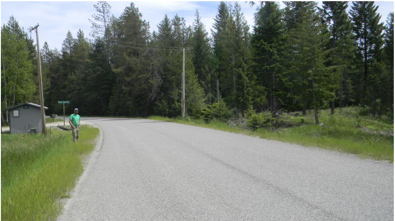
Figure 25. Photograph of the Cabinet Mountain Water District Project area taken at the existing Highland Meadows Booster Station. Highland Flats Road is in the foreground. The new booster station will be constructed in this vicinity; the three potential locations are in the alfalfa field to the left, in the trees in the left background, or to the right of Highland Flats Road. The view is to the east.
