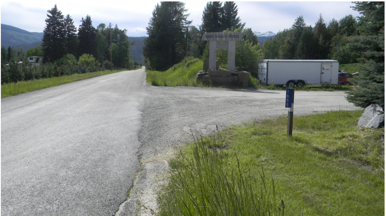
Figure 39. Photograph of the Cabinet Mountain Water District Project taken along the waterline route between the Highland Booster Station and access road to the new Highland Tank. Highland Flats Road is at the left. The view is to the west.
