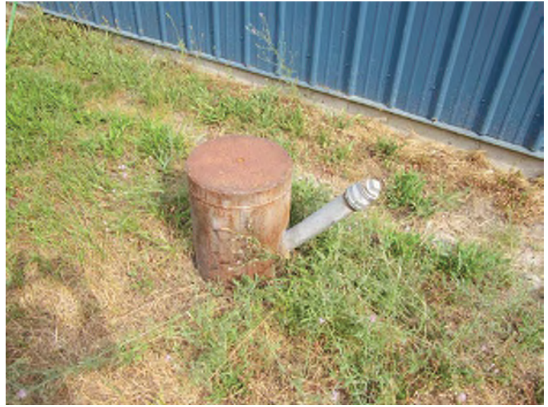
Photograph 6: Test well (capped)
