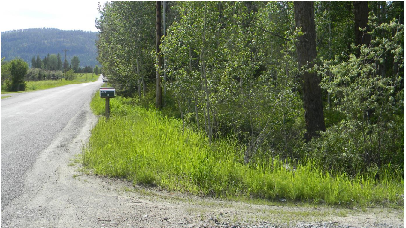
Figure 40. Photograph of the Cabinet Mountain Water District Project taken along the waterline route between the Highland Booster Station and the access road to the new Highland Tank. Highland Flats Road is at the left. The view is to the west.
