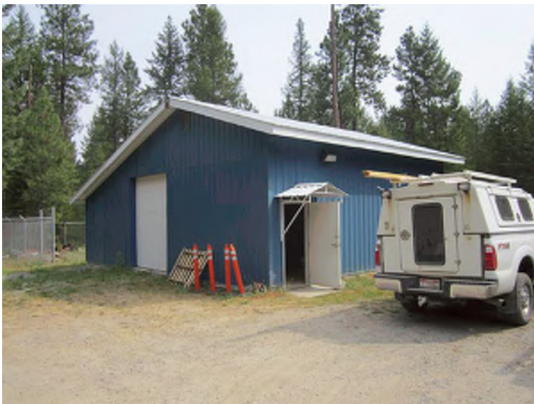
Photograph 23: Well 1 and 2 building
