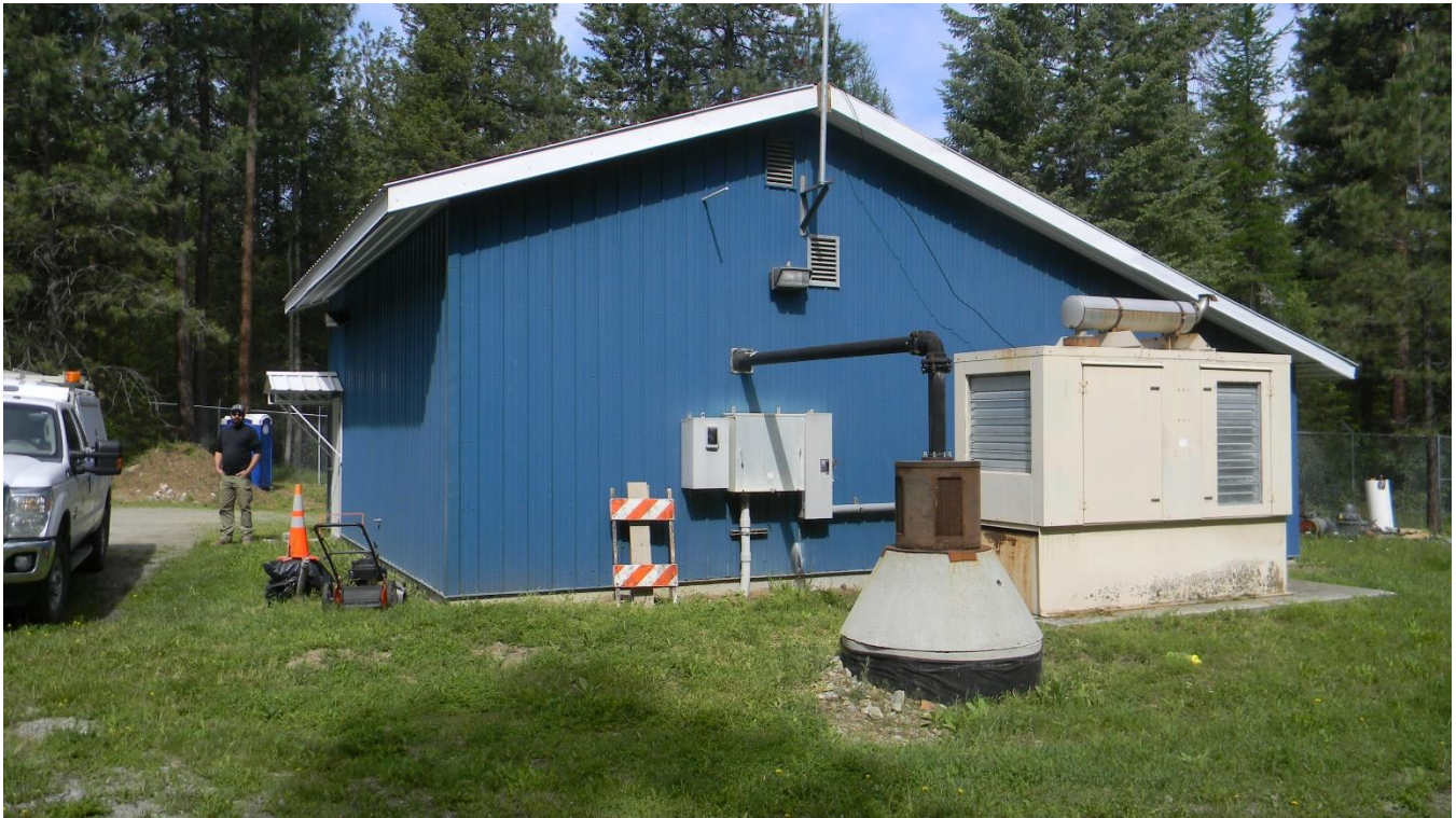
Figure 8. Photograph of the Cabinet Mountain Water District Project area taken at the existing Crossport wellhouse/office building. The new well will be located in the vicinity of Jeremy Davy who is standing to the left of the building. The view is to the west.
