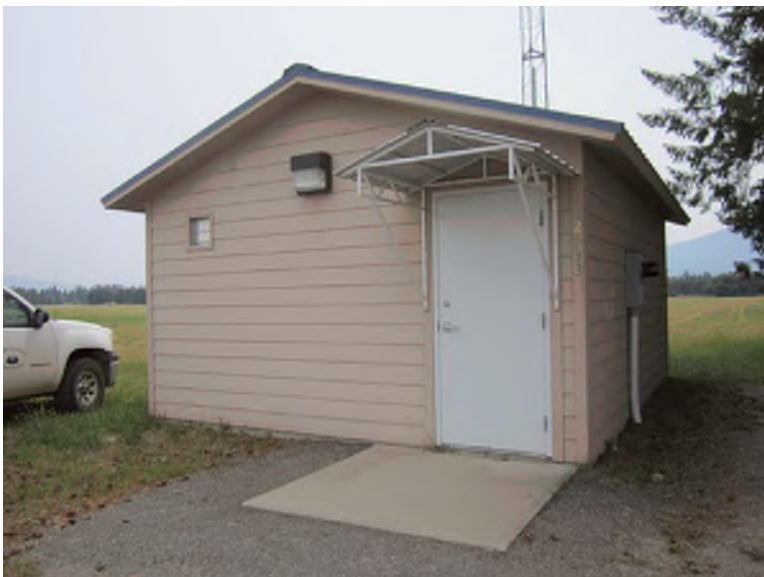
Photograph 47: Four Corners booster station
