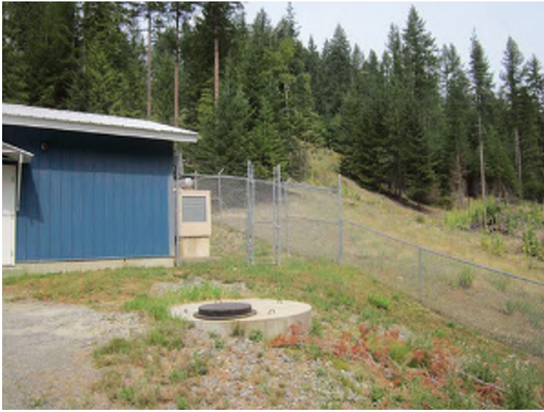
Photograph 25: Parker Canyon diesel generator
