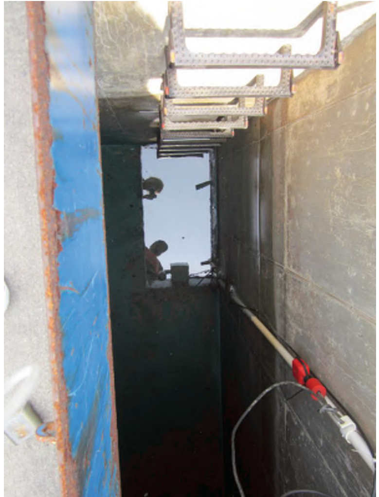
Photograph 50: Black Mountain reservoir interior
