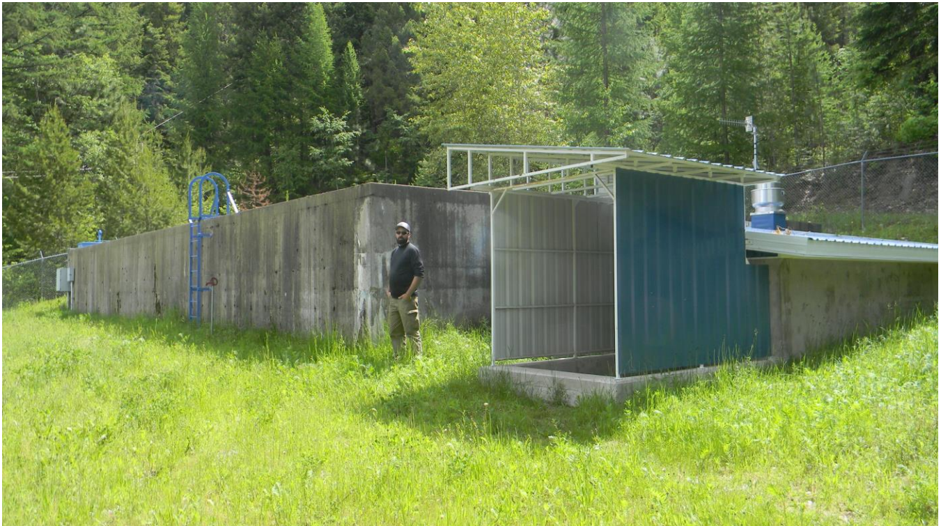
Figure 17. Photograph of the Cabinet Mountain Water District Project area taken at the existing Black Mountain Tank and Booster Station. Jeremy Davy is standing near the northwest corner of the tank. The view is to the southeast.
