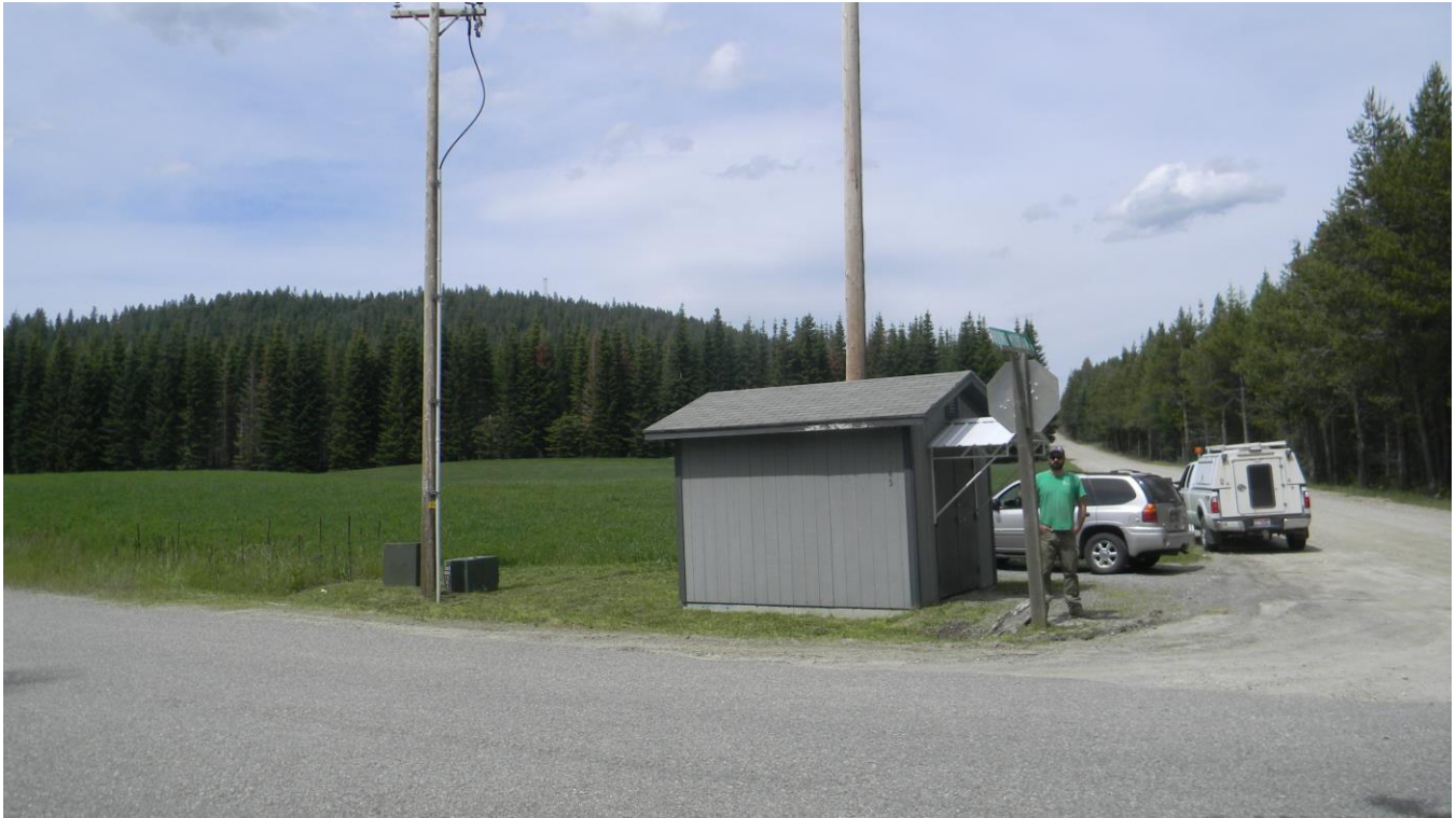
Figure 24. Photograph of the Cabinet Mountain Water District Project area taken at the southeast corner of the existing Highland Meadows Booster Station. The new booster station will be constructed in this vicinity. Highland Flats Road is in the foreground; Round Mountain Road is at the right. The view is to the north.
