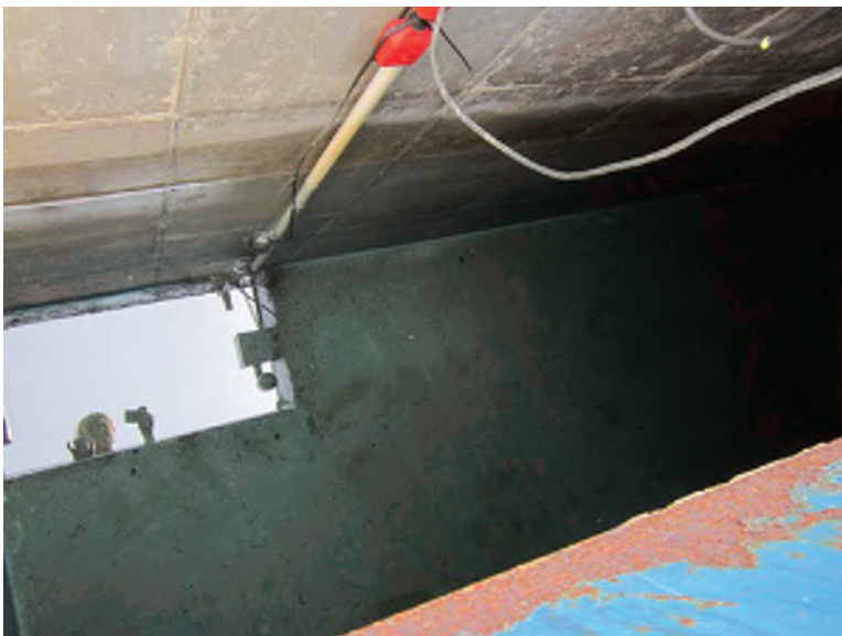
Photograph 51: Black Mountain reservoir interior
