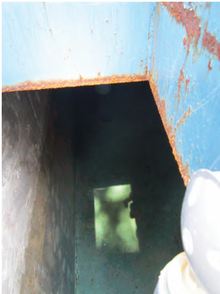
Photograph 82: Naples tank interior
