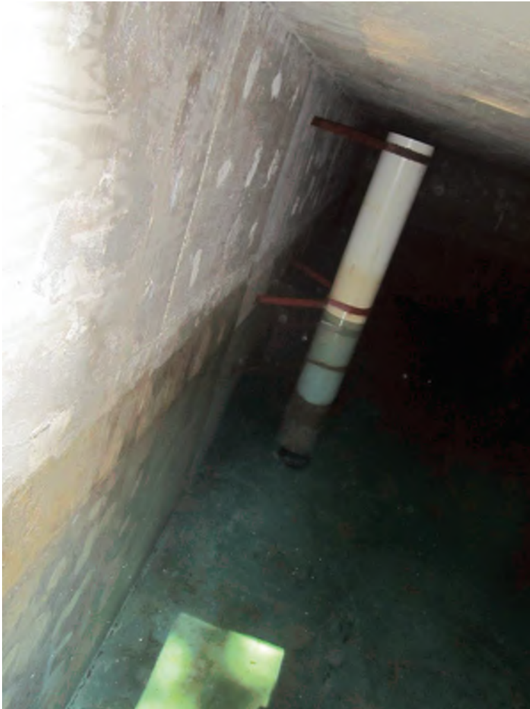
Photograph 85: Naples tank overflow
