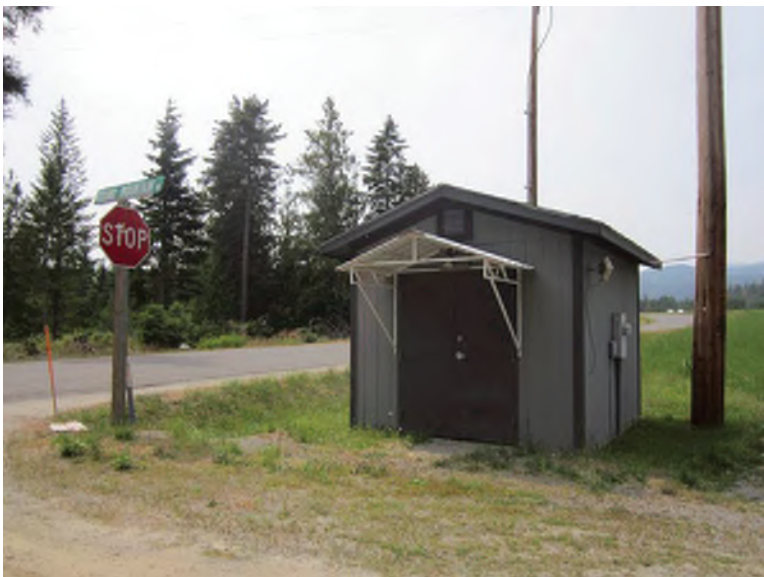
Photograph 99: Highland Flats booster station building
