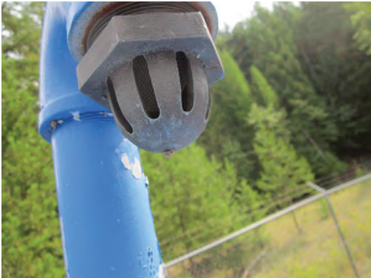
Photograph 55: Black Mountain reservoir vent w 24-mesh screen
