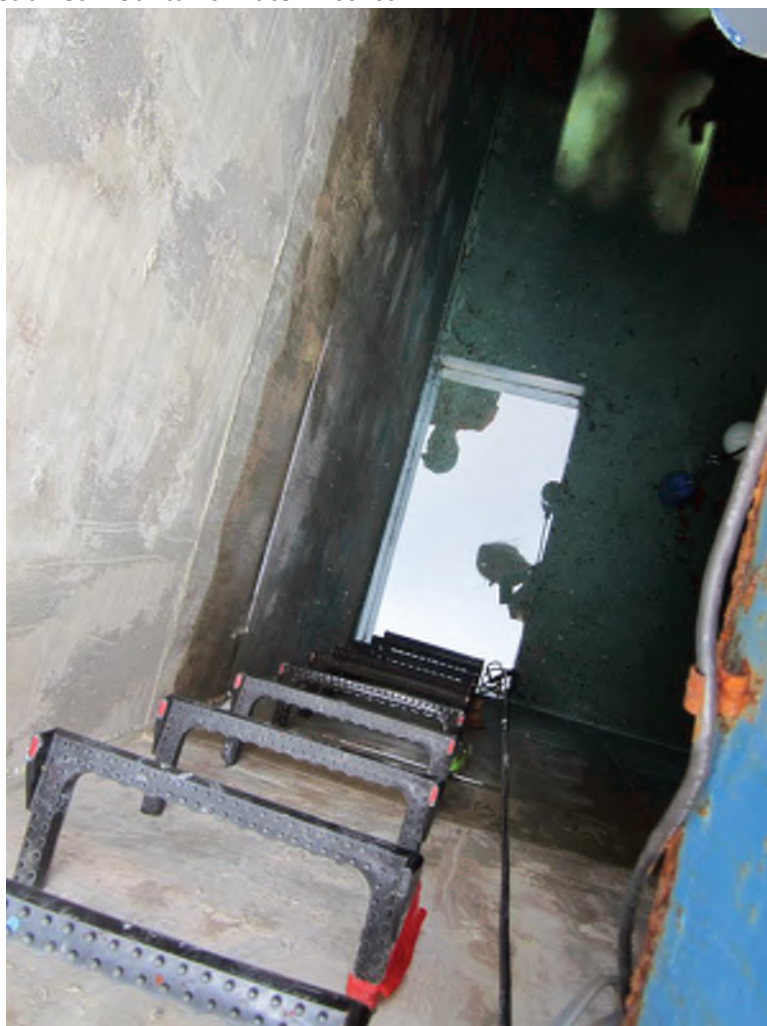
Photograph 84: Naples tank interior
