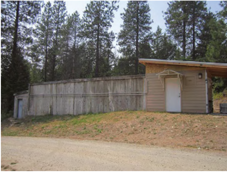
Photograph 73: Naples tank and booster station
