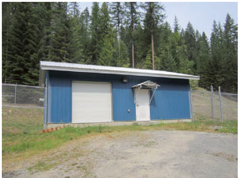
Photograph 24: Parker Canyon booster station
