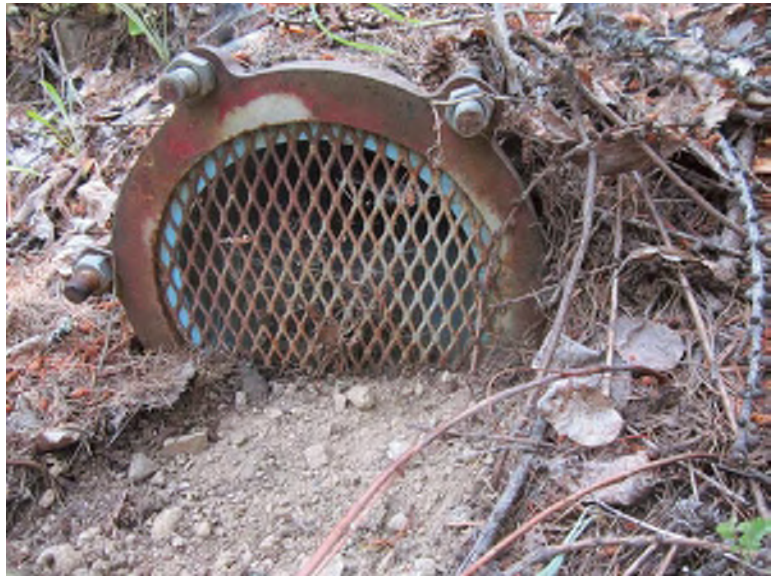
Photograph 68: Black Mountain reservoir screened drain
